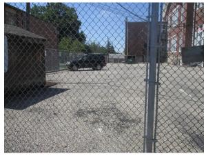
Erosion is evident in the asphalt of the courtyard. The parking spaces can be replaced with porous pavement to capture, treat, and infiltrate roof and pavement runoff. A preliminary soil assessment suggests that the soils have suitable drainage characteristics for green infrastructure.
