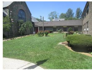
Rain gardens adjacent to the building can capture, treat, and infiltrate runoff from the roof when their respective downspouts are disconnected. A section of the parking lot along the property where flooding is an issue can be replaced with porous asphalt to capture runoff. A preliminary soil assessment suggests that the soils have suitable drainage characteristics for green infrastructure.
