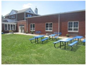
Multiple downspouts along the southern side of the building can be disconnected to redirect rainwater to two rain gardens. Rain gardens can be used to capture, treat, and infiltrate roof runoff. A preliminary soil assessment suggests that the soils have suitable drainage characteristics for green infrastructure.
