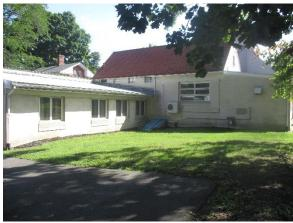
Rain gardens adjacent to the buildings can capture, treat, and infiltrate roof runoff. Existing downspouts on the western building can be disconnected and rerouted to the rain garden. The downspout on the eastern building is already disconnected. A preliminary soil assessment suggests that the soils have suitable drainage characteristics for green infrastructure.
