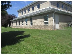
Downspouts originating from the roofs of the two buildings can be disconnected and rerouted to two rain gardens to capture, treat, and infiltrate roof runoff. A preliminary soil assessment suggests that the soils have suitable drainage characteristics for green infrastructure.
